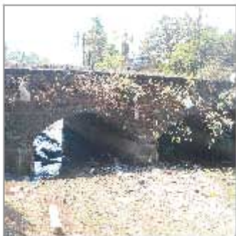
Pantawane Bridge, Ratnagiri, Nagar Parishad, Ratnagiri.
